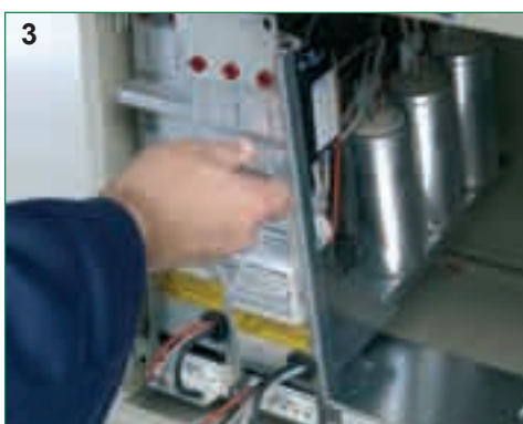
Remove the module to be replaced
