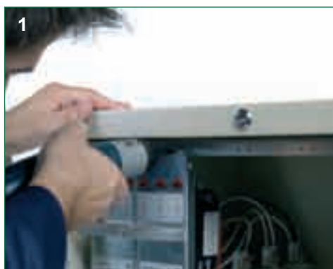
Withdraw 2 fixing screws
